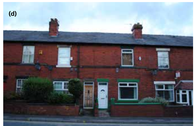
Figure 1: Examples of typical wall construction types to which solid wall insulation may be applied: (a) brick solid wall, (b) stone solid wall, (c) system build (BISF steel frame), (d) narrow cavity wall
