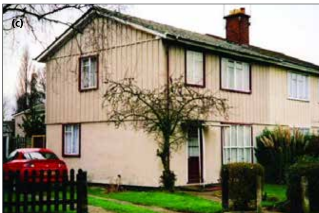
Figure 1: Examples of typical wall construction types to which solid wall insulation may be applied: (a) brick solid wall, (b) stone solid wall, (c) system build (BISF steel frame), (d) narrow cavity wall
