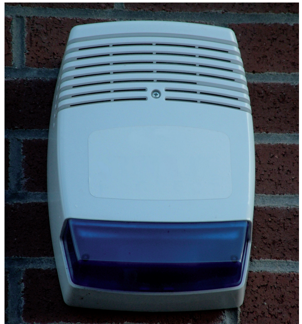
Figure 1: Intruder alarm external sounder
