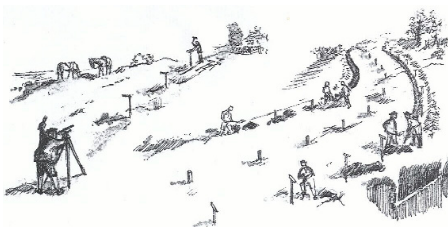
Figure 1.7 Marking out the construction levels for a canal. First, level pegs were driven, with crosspieces indicating the depths to be dug. Opposite each one, a peg was driven to mark the centreline of the canal. Holes were then dug at each side to indicate the course and width of the canal channel. These were joined as trenches to define the canal banks and the channel excavated (Paget-Tomlinson, 1996)
