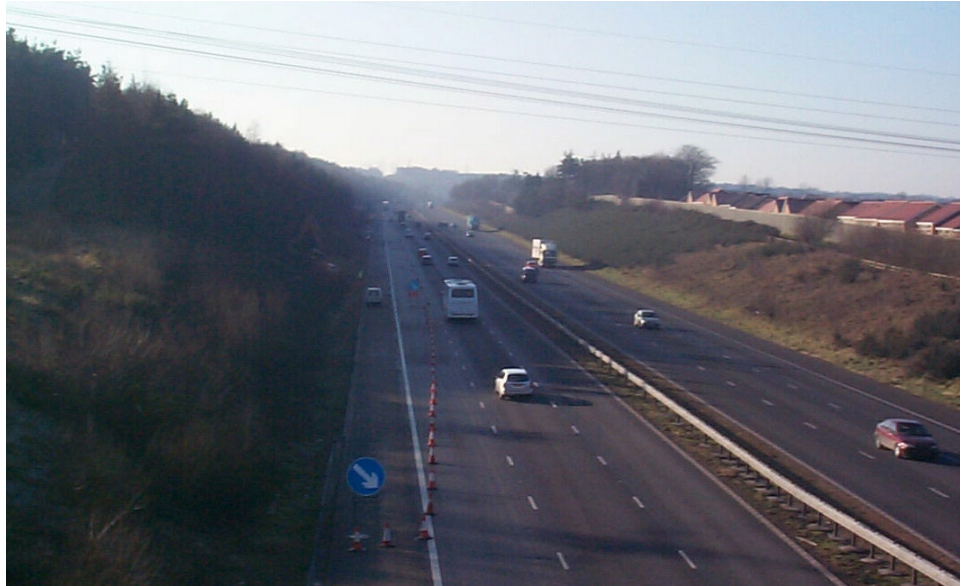
Figure 1.5 Example of an infrastructure cutting
