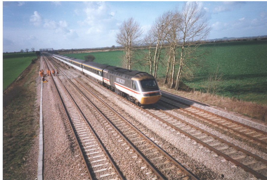
Figure 1.1 Railway embankment. Poor compaction and steep slopes are characteristic of this type of embankment
