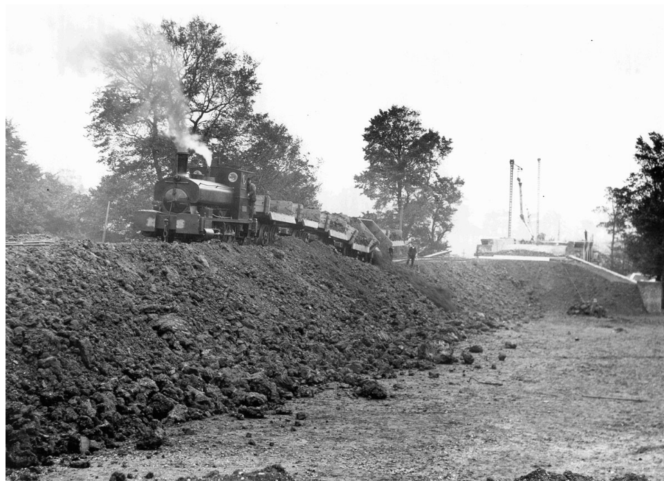
Figure 1.9 LUL Edgware extension construction in 1922 showing side-tipping trucks depositing clay onto the slope of an embankment as part of the filling process (courtesy London Transport Museum)
