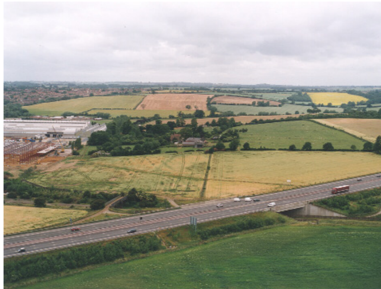
Figure 1.2 Highway embankment. Construction and design is to modern standards with adequate compaction and flatter slopes (courtesy Adkins Photography)
