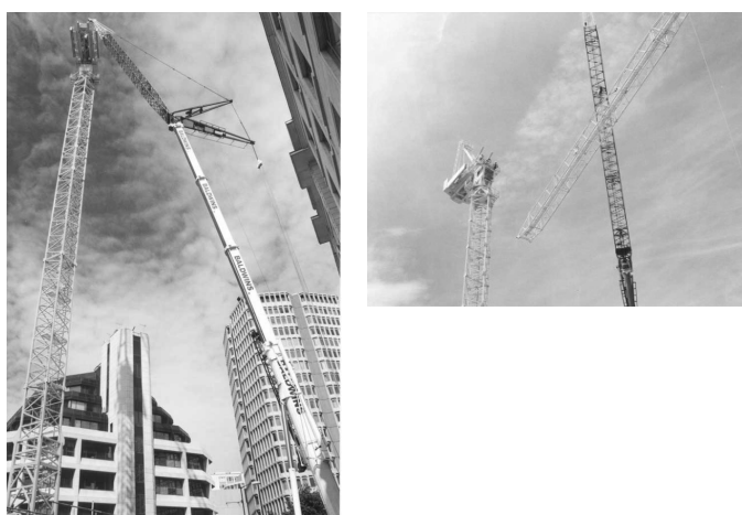
Figure 1.1 Tower crane erection
