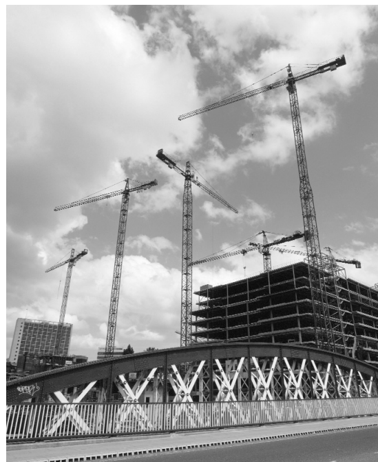
Figure 1.8 Tower cranes on site
