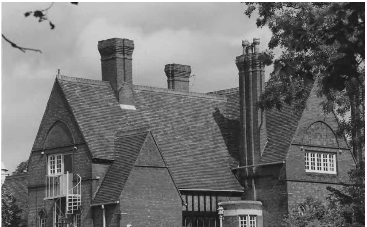
Figure 3.1 This steeply pitched plain tiled roof was built in 1880 but re-covered after bomb damage in the 1939–45 war
