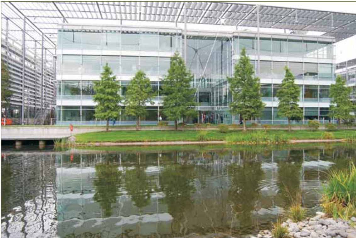
Figure 1.1 Recently planted large species trees incorporated into the recent commercial development at Chiswick Park, London
