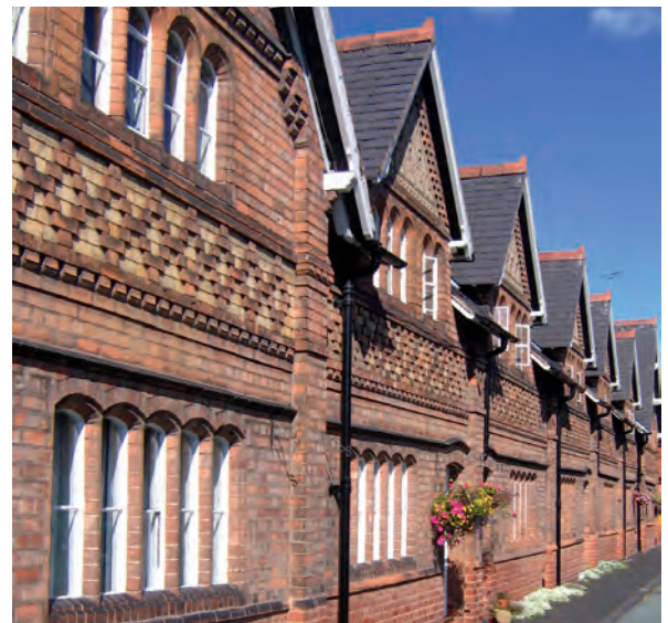
Figure 1: Intricate masonry façade of a Victorian building employing 'traditional' forms of construction
