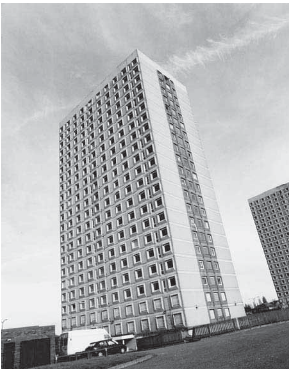
Figure 1: Bison LPS dwelling block (courtesy Sandwell Metropolitan Borough Council)
