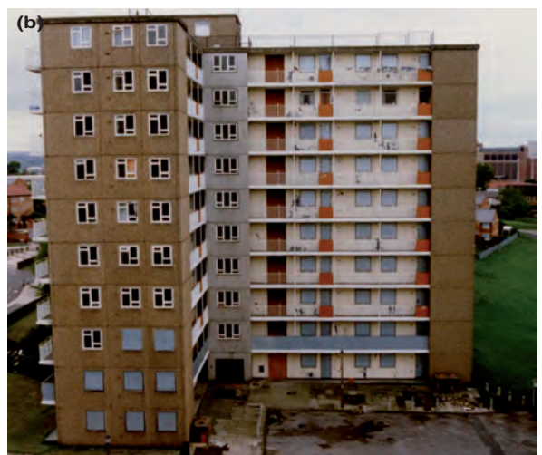
Examples of the large panel system (LPS) built dwelling blocks load-tested by BRE: (a) a Bison LPS dwelling block, (b) a Reema Conclad LPS dwelling block
