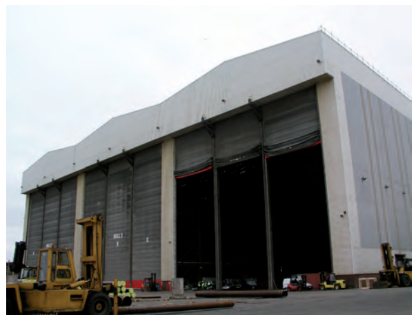
Figure 1: Smoke pellet burn test under way in 43.5 m high hangar
