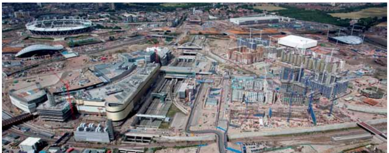
Figure 1: Aerial view of the 2012 Olympic Park and Olympic and Paralympic Village during construction
