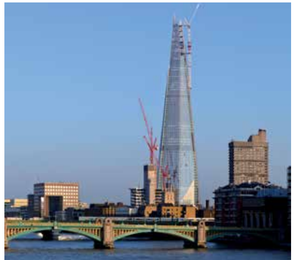
Figure 1: A tall modern building
