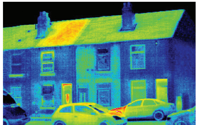
Figure 1: A thermogram of a street visualising heat in the roof of one of the terrace of houses (suggesting poor or no loft insulation), the same property's door and the engine of a recently parked car
