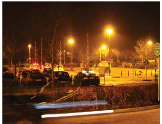
Figure 1: Car park lanterns giving upward and sideways spill light as well as useful downward light
