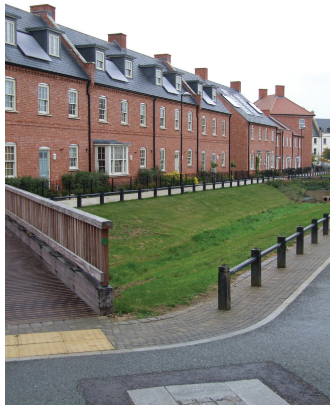
Figure 1: An example of a swale introduced into a housing estate in Upton, Northamptonshire
