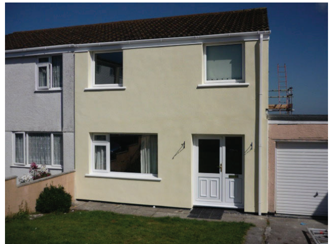
External wall insulation applied to a timber hybrid dwelling (© Ocean Services)
