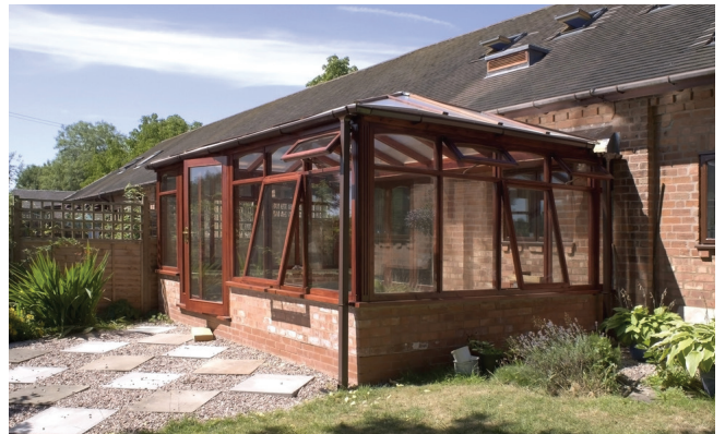
Figure 1: A typical conservatory to an existing property
