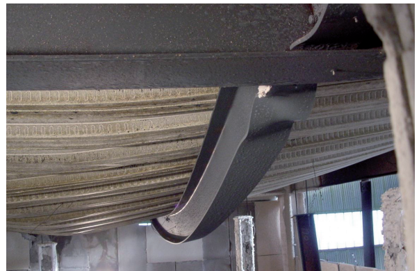
Figure 1: Damage to unprotected steelwork following a large-scale fire test
