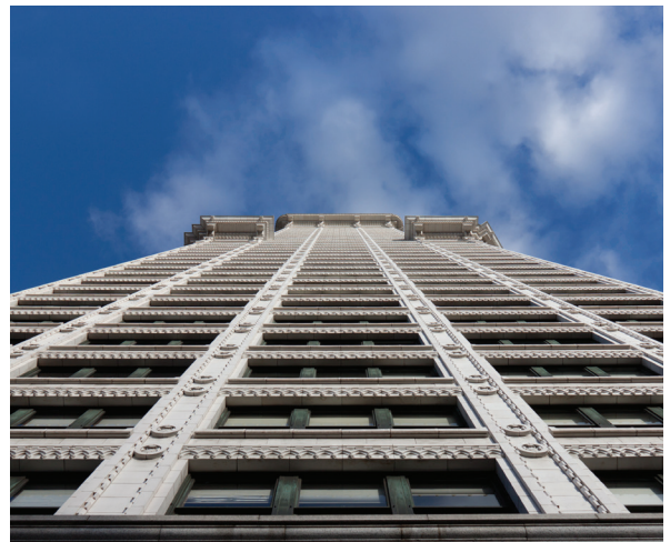
Figure 1: Looking up the facade of a terracotta office building
