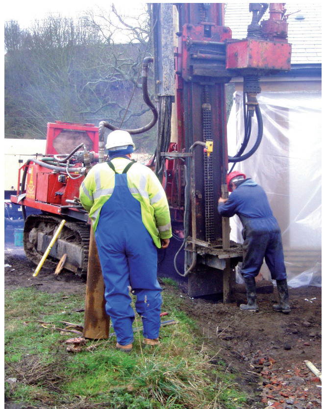
Figure 1: Installing a heat exchanger for a ground source heat pump
