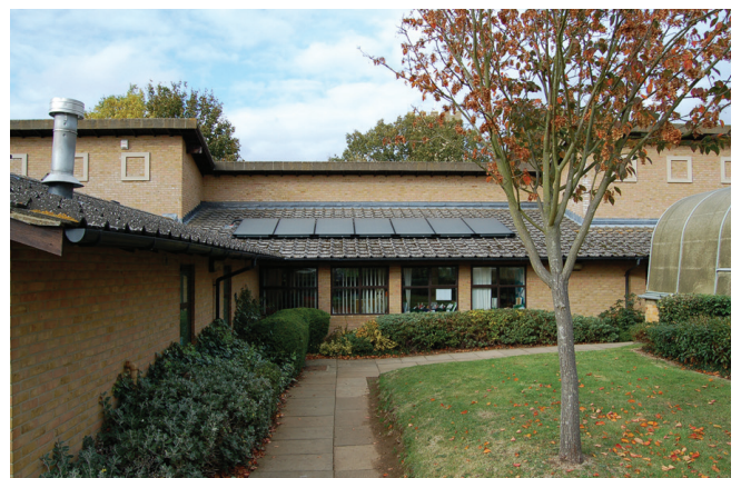
Figure 1: A solar thermal installation
